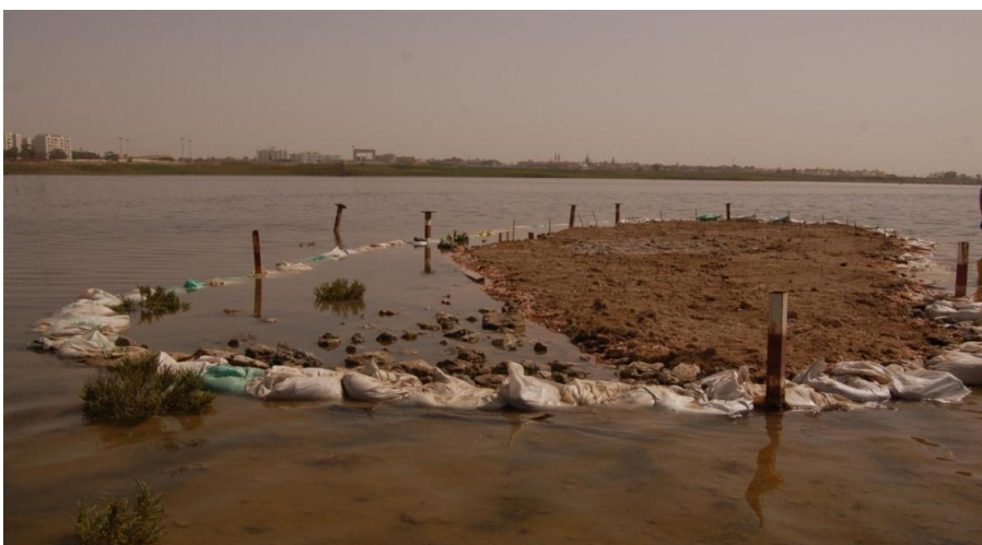
The islet after restoration in April 2012
