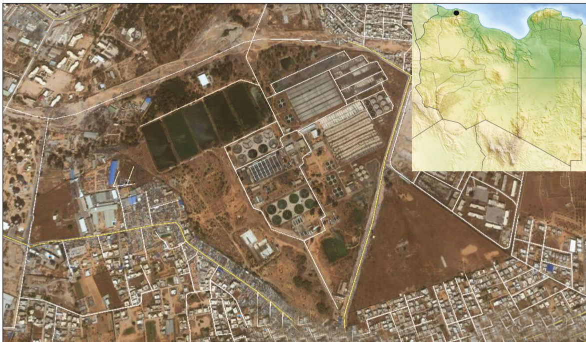
Figure 1. Study area: Al-Hadba station for sewage treatment.
